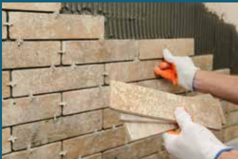
Internal tiling on walls
