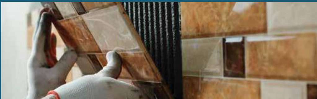
Tile repairs and rehabilitation works
