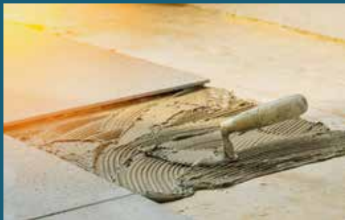
Internal tiling on floors
